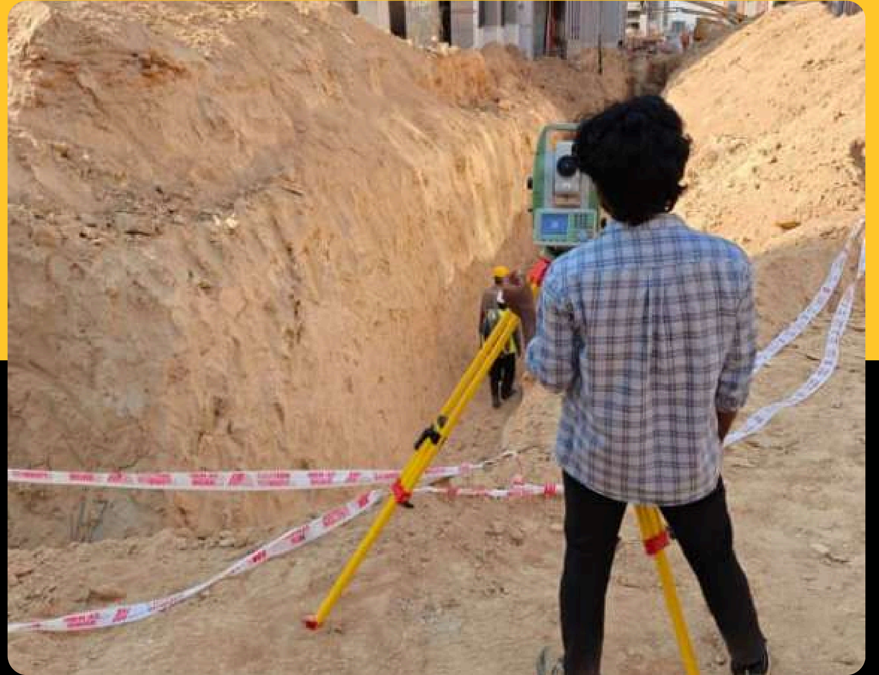
Marking chamber points and elevations from surveyor
